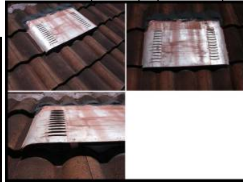
Attic ventilation has exposed louvers that is allowing moisture penetration. Also, the vent does not provide proper rodent protection from attic entry.
